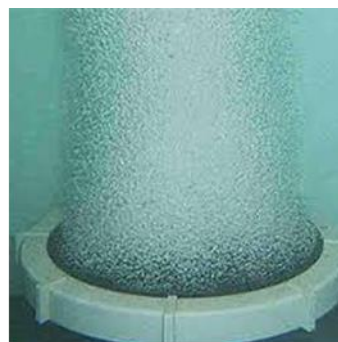
Figure 19: Coarse Bubble Air Diffusion Systems Source: southern cogen systems PVT. LTD.
