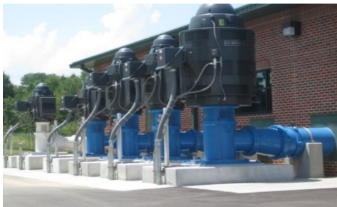
Figure 8: 21 MGD Finished Water Pumping Station Albertville, AL, USA (Source: KREBS Engineering)
