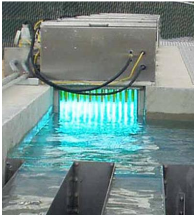
Figure 5 UV Disinfection System (source American Air and Water)
