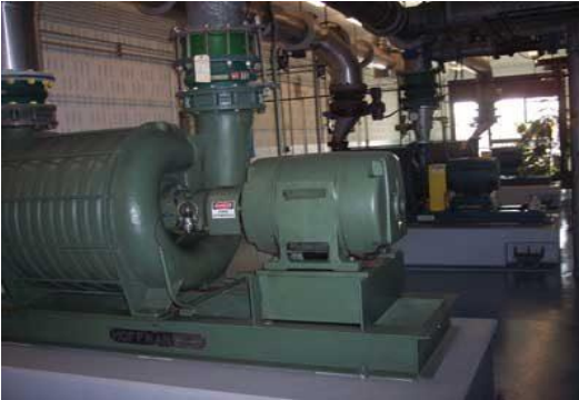
Figure 16: Multistage Centrifugal Blower (Source: waterworld.com)
