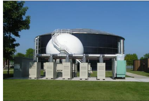
Figure 24: Micro Turbines at the Sheboygan WWTP (Source: City of Sheboygan, WI website)
