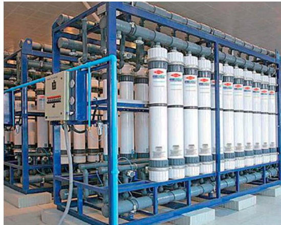
Figure 6 Membrane Filtration (source Arifiks Engineering)
