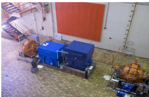
Figure 9: 2000hp, 90ML/d High Lift Pump Edmonton, AB, E.L. Smith Water Treatment Plant (Source: Edmonton Journal)
