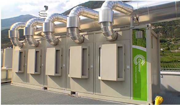
Figure 23: Micro Turbine Power Generators (Source: decentralizedenergy.com)
