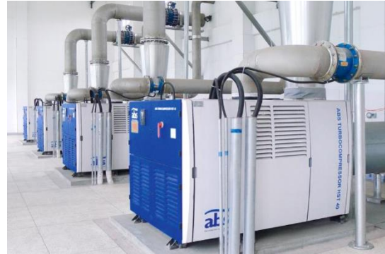
Figure 17: Turbo Blower (Source: Sulzer.com)
