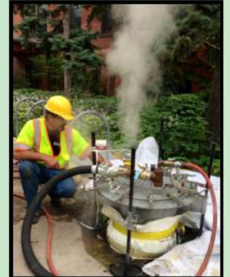
Pressurized Heat Curing
