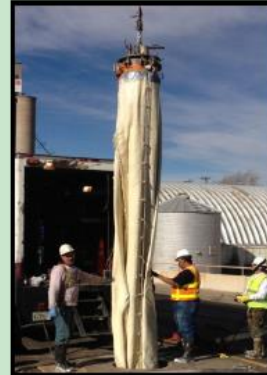
Lowering into Structure
