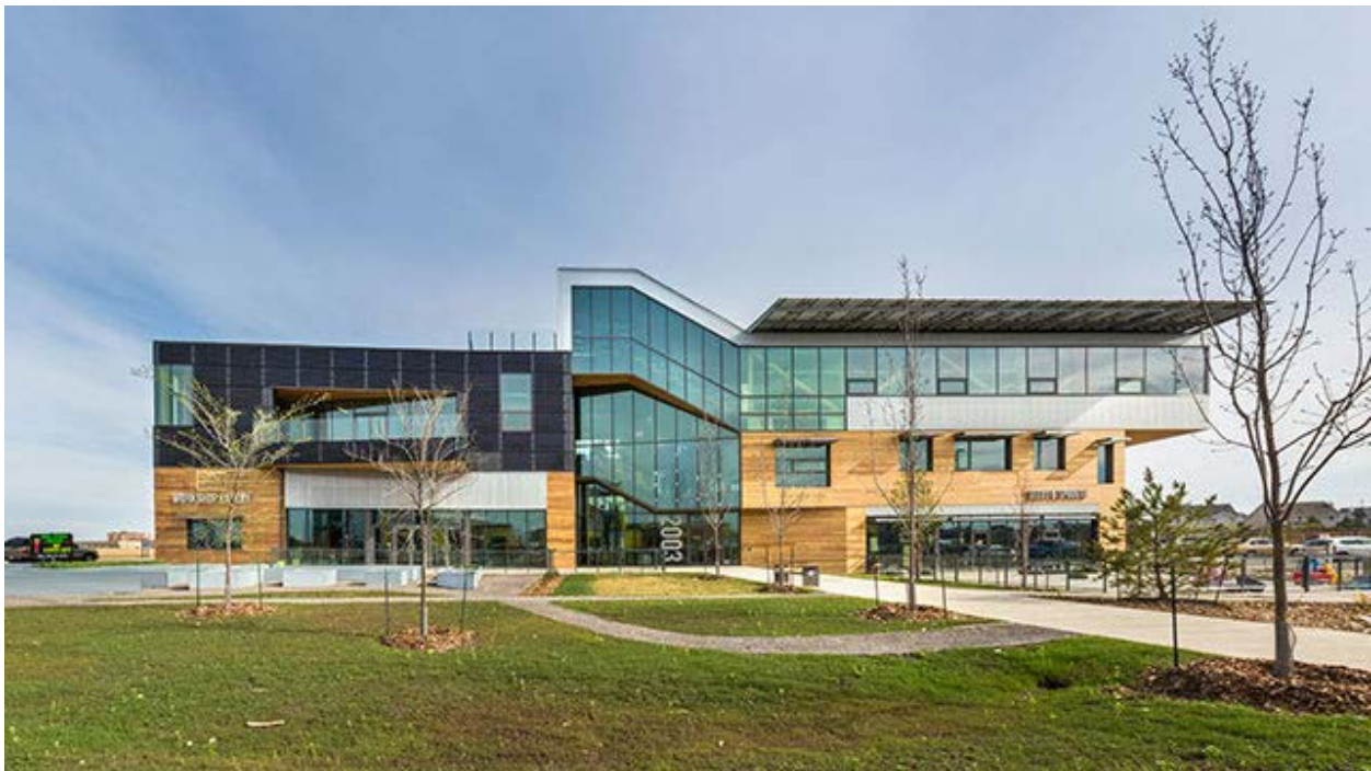
Edmonton's Mosaic Centre utilizes a geo-exchange system of 32 boreholes of 70m depth to provide heating and cooling to the building.
