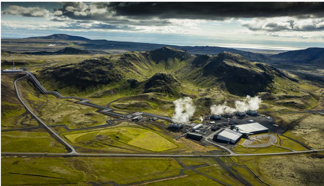
Hellisheði Geothermal Power Plant, Iceland. 303MW electrical capacity and up to 400MW thermal capacity from 500l/s steam at 180°C.
