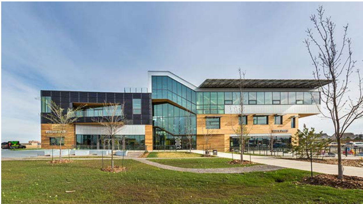
Edmonton's Mosaic Centre utilizes a geo-exchange system of 32 boreholes of 70m depth to provide heating and cooling to the building.
